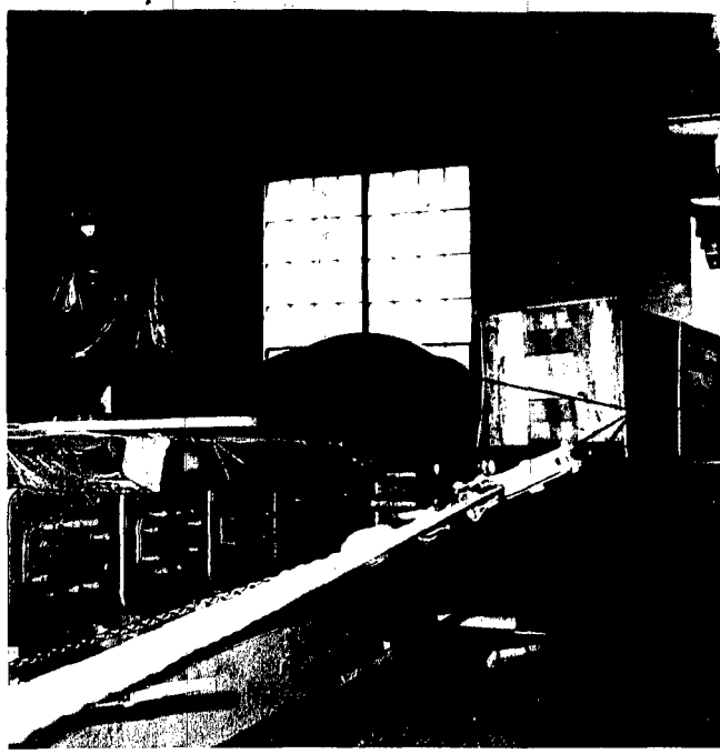
BIG MOVE. The 16,000-pound crankshaft for the Municipal power plant's Worthington generator engine was inched into the building and onto the engine base last week as work continued to put the big engine back into operation. The shaft will be set in place. Plant Superintendent Norbert
